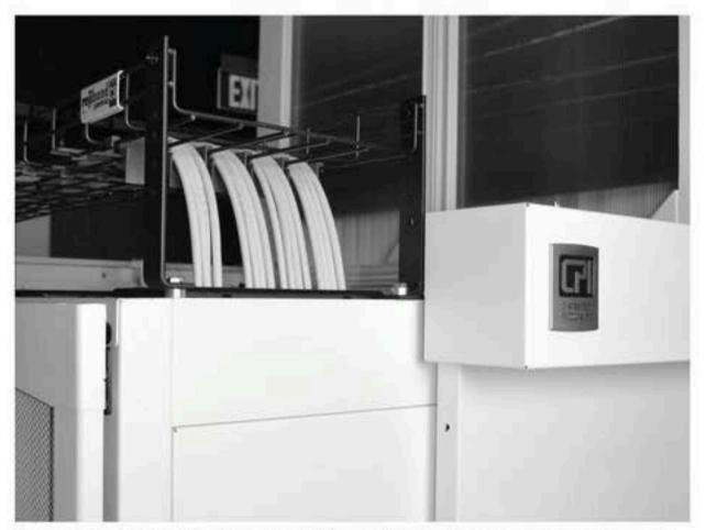
The wire mesh cable tray is another TR essential, as it can be supported from the wall, ceiling, floor or from the tops of open racks.
