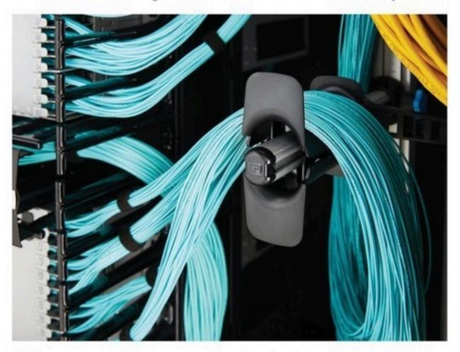
Cable management solutions are evolving from simple troughs that hold cable bundles in place to mechanical systems that can now adjust to optimize cable support exactly where needed.
