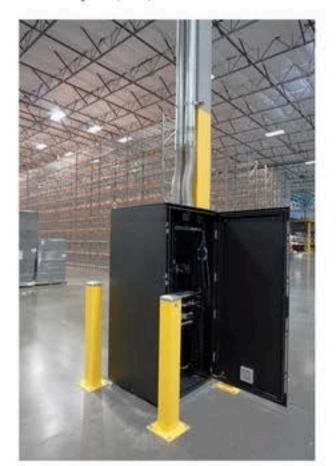
Advanced factories, warehouses and outdoor locations require environmentally rated enclosures and appropriate cooling and power accessories to ensure they can function as the TR itself.
