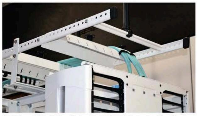
Installations with multiple cable drops greatly benefit from adjustable cable runways, which offer movable cross members, allowing for maximum flexibility.
