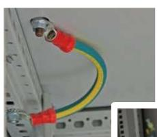
When deploying enclosures, it is important to select grounding and bonding wires that meet the application's required amperage. Bond the top, side panels and the doors to the enclosure frame.
