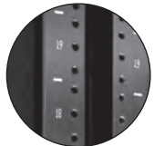
U marks simplify equipment installation
