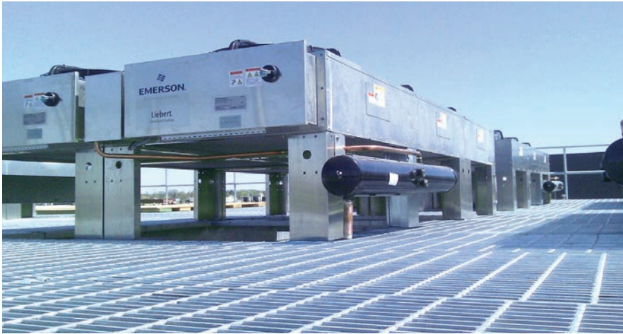
The Primus data centre has been awarded Uptime Institute's prestigious Tier III Certification for Design Documents.
