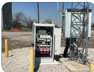
NEMA-rated industrial enclosures to protect equipment outdoors
