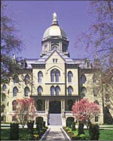
University of Notre Dame faces the challenge of a continually growing and changing campus.
