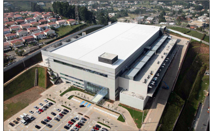
Telefônica Vivo planned its state-of-the-art data center to support the evolution of technology for the next 10 years or more.
