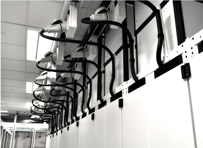
CPI manufactured custom cable openings into the cabinets to fit UF Health Shands' unique design.
