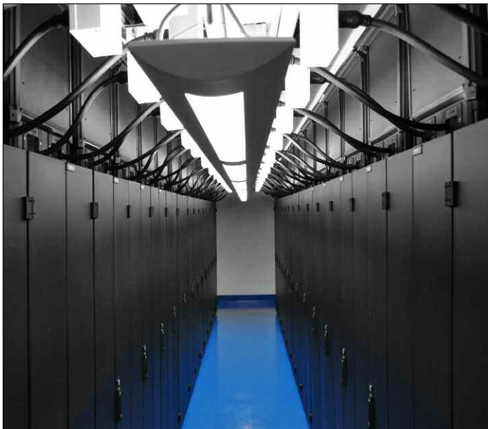
CPI's Passive Cooling isolates and segregates hot air while allowing for overhead power busway.
