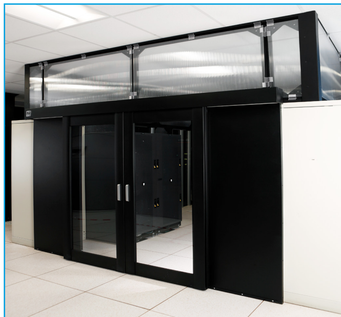
Sliding aisle containment doors seal the ends of the aisles without adding any additional clearance requirements. This solution integrates with perimeter cooling, provides immediate improved cooling efficiency and is compatible with economization methods.
