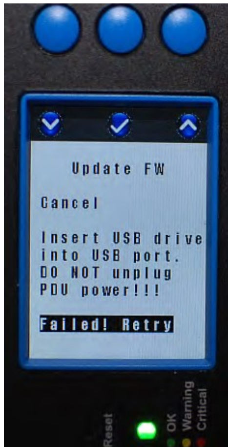
Sample of Failed updating – (below)
