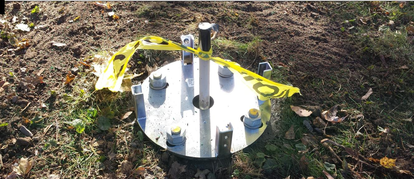
After the concrete has set, remove the bolt positioner board. Leave the lower nuts and washers in place for anchor base installation. Place the anchor base over the nuts. Level the anchor base, then fasten with another set of nuts and washers. Pull the data and power cables through the conduit.
