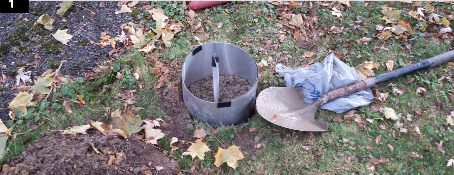
Dig a hole at least 11.5" diameter minimum in the desired location for the assembly. The hole depth is determined by the frostline of the installation location. 30" is the minimum recommended. The sidewalls must be flush and plumb. Uneven sidewalls can cause the foundation to fail or tilt.
