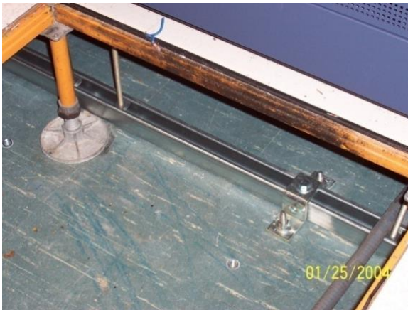
Subfloor bracing.
