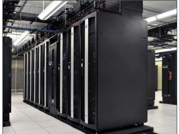
Rows of F-Series TeraFrame® Cabinets with Vertical Exhaust Ducts help the State of Montana maintain a PUE of less than 1.1 by keeping hot exhaust air isolated in the cabinet and separate from the room.
