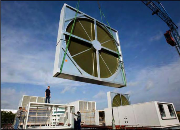
The KyotoCooling® wheel is installed at the State of Montana data center, making it the first in the US to deploy this emerging technology.
