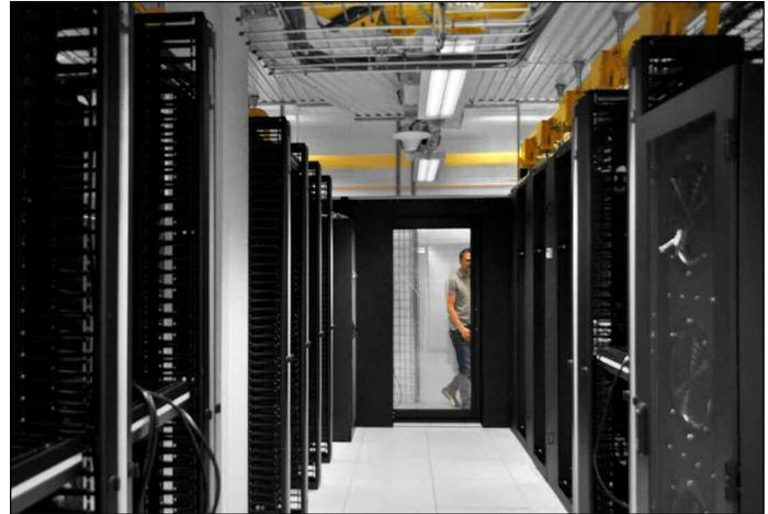
Open Architecture design supports Hot Aisle Containment and allows for more equipment.
